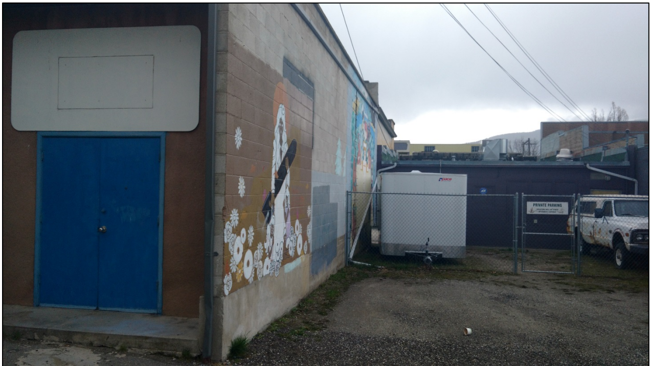
Figure 7: North Building Face (from the lane)
