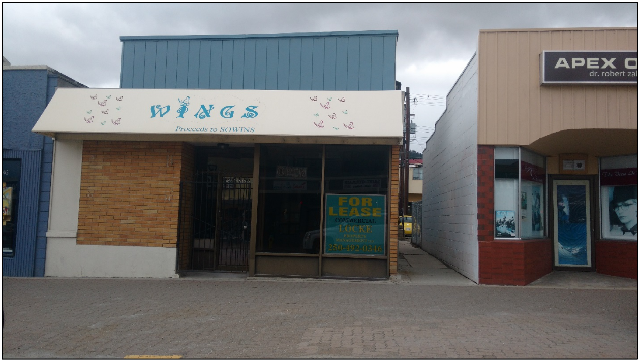
Figure 4: West View (from Main Street)
